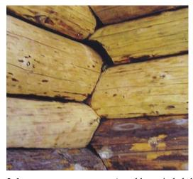
Figure 2. Incorrect corner structure (roughly encircled shapes)
