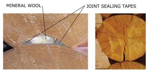
Figure 3. Examples of correct and incorrect groove type
