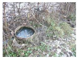
Photo 4. Malfunctioning of the drainage pipeworks due to the mass movement
