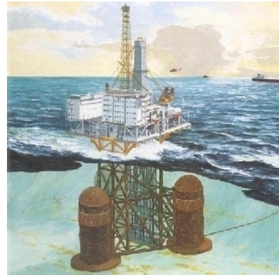
Fig.2 Maureen steel gravity-based platform, U.K.
