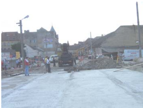
Photo 3 - Equalization concrete layer
