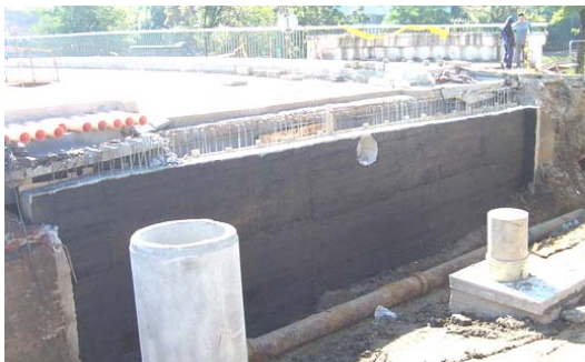
Photo 5 - New retaining wall
