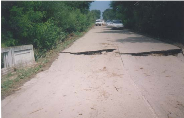
Figure 5. The earthwork creeping behind the abutment
