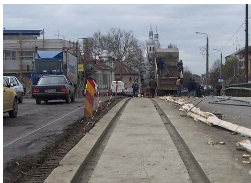
Photo 13 – ICOSIT System on the Decebal Bridge and on the M. Viteazu Bridge
