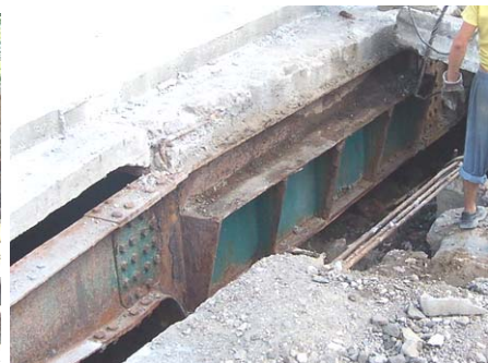
Photo 6 - The steel structure corrosion
