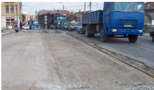
Photo 9 - Cleaned concrete plate
