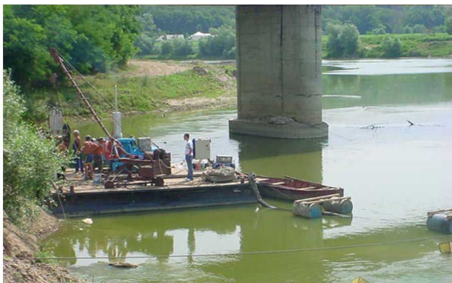
Figure 8. The bridge from Ion Creangă over Siret River – rehabilitation works and securitization of the pile no. 10, after the scour phenomena manifestation
