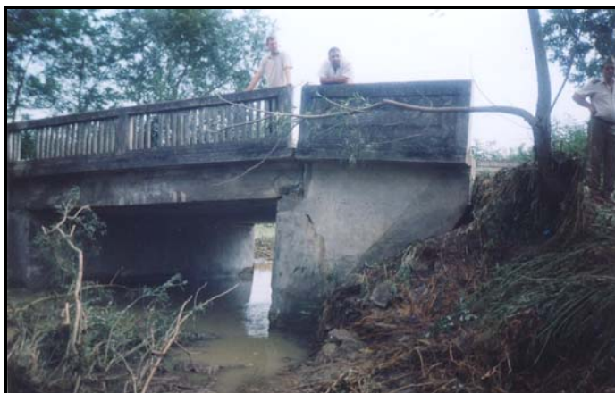
Figure 4. Abutment displacement from the initial position with scour of the con's quarter.
