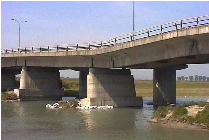
Figure 1. Pier no 6 of the bridge crossing Moldova River, from Roman, displaced due to an erosion process.
