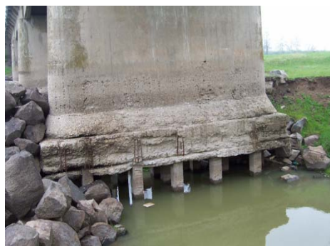
Fig.3 Pier founded on piles
