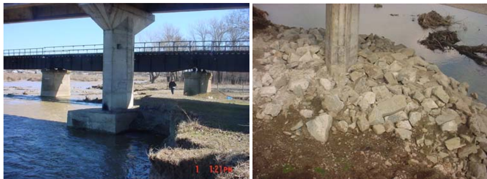
Figure 7. The Dornești Bridge: the change in plan of the water course lay-out, before and after rehabilitation
