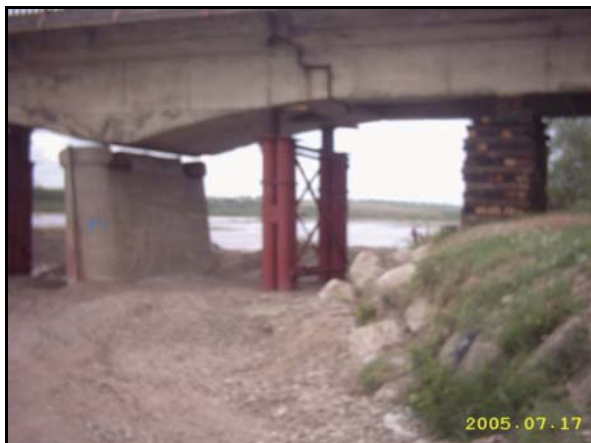
Fig. 8. Repairs at Tupilați bridge
