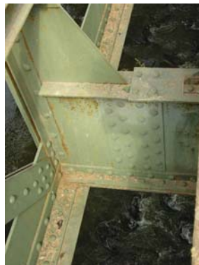
Figure 4. Detail of the connection cross girders-main girders
