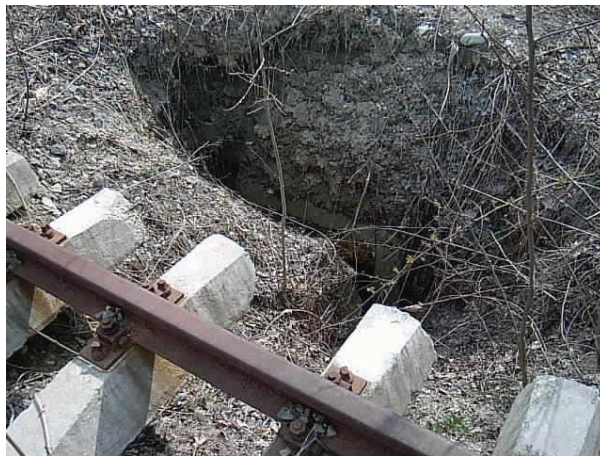
Photo 1 Embankment's Sliding
