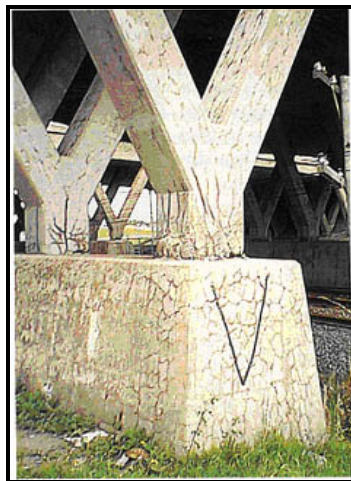
Figure 9. Network cracking (Source: http://www.filer.case.edu )
