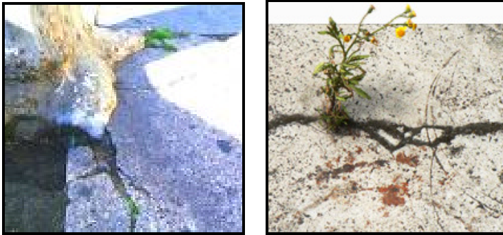
Figure 16. Environmental cracks (Source: http://www.ewhow.com ; http://www.imagination.lancaster.ac.uk )
