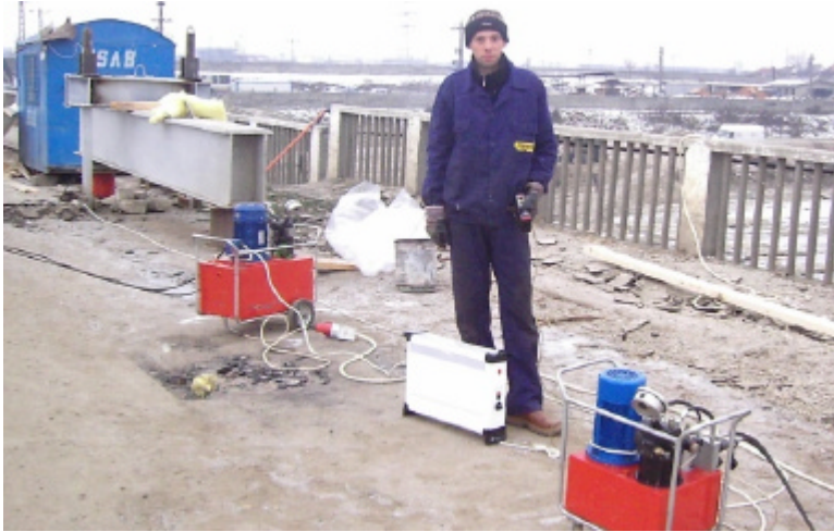
Photo 27. The installation of the hydraulic and electrical equipment
