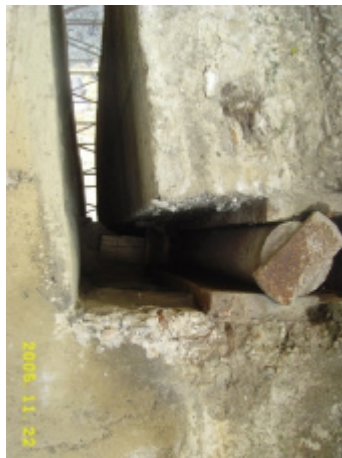
Photo 14. Degradations of the mobile-bearing devices
