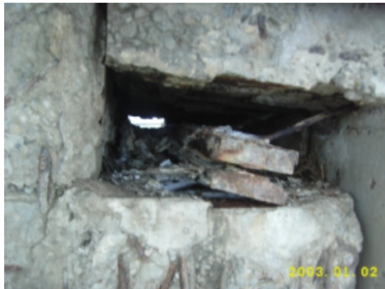
Photo 16. Degradations of the fixed-bearing devices (detected after the lifting of the deck)
