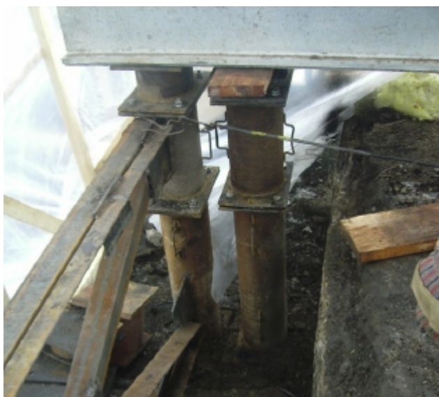
Photo 31. The final bearing of the lifting beam
