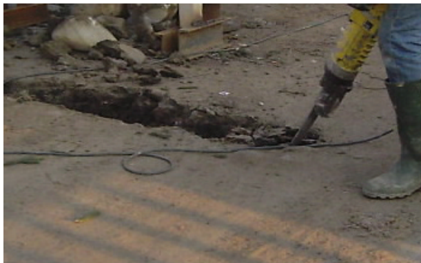
Photo 25. The disposing of the covering devices of the expansion joints
