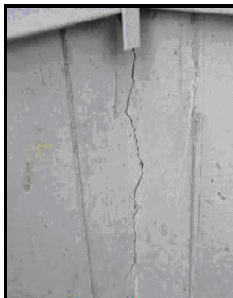
Figure 14. Shrinkage cracks (Source: http://www.inspect-ny.com )
