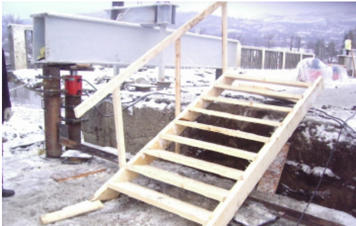
Photo 29. Horizontal bracing on the lower side of the steel supports
