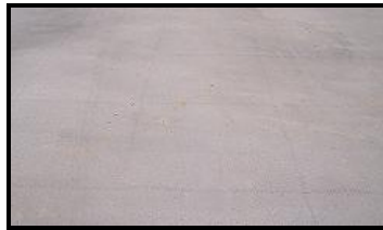
Figure 5. Drying shrinkage cracking (Source: http://www.members.optusnet.com.au )
