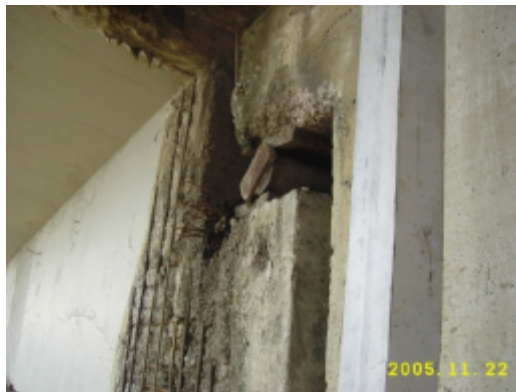
Photo 13. Concrete degradation in the bearings area
