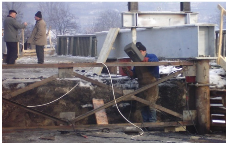
Photo 30. The cross-bracing of the steel supports
