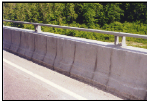
Figure 13. Temperature cracks (Source: http://www.irc.nrc-cnrc.gc.ca )
