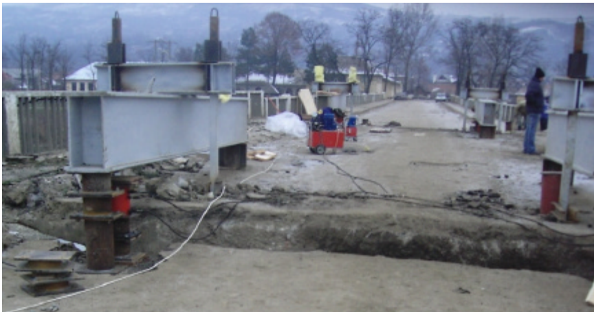
Photo 28. The deck lifted with h=40\text{cm}
