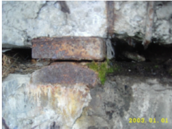
Photo 15. Degradations of the fixed-bearing devices
