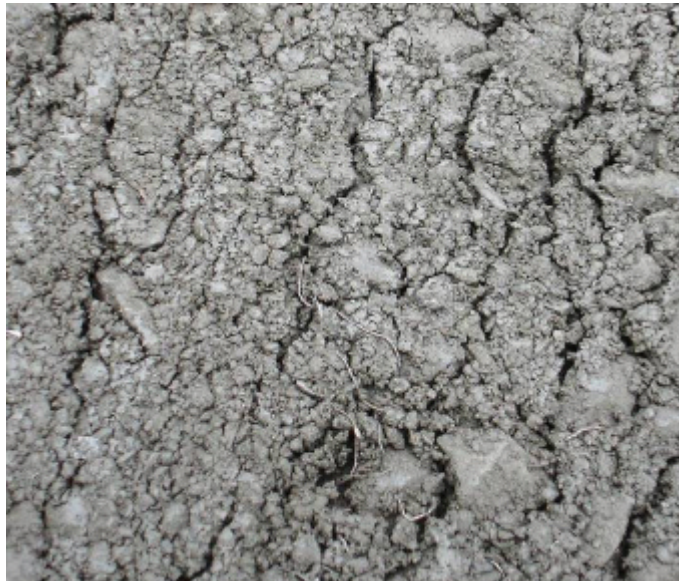
Figure 6 – Surface of SFR-RCC pavement following paver compaction
