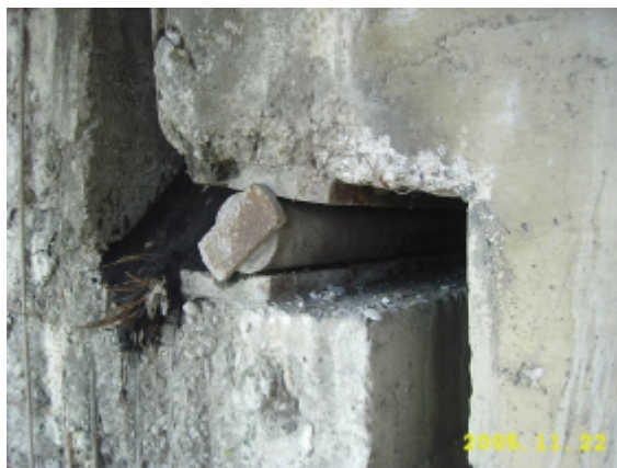
Photo 17. Degradations of the concrete in the mobile-bearing devices area, degradations of the bearing device elements and the blockage of the construction joint by aggregates from the road coating.
