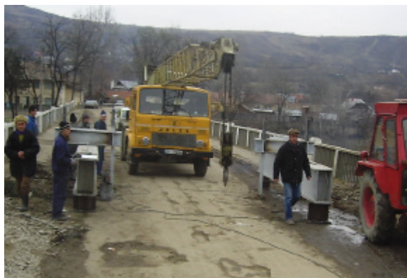
Photo 26. The installation of the lifting device
