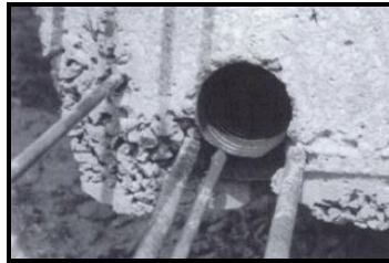
Figure 8. Honeycomb cracking (Source: Handbook of concrete bridge management De Jorge de Brito)
