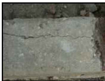
Figure 6. Corrosion crack (Source: http://www.upload.wikimedia.org )
