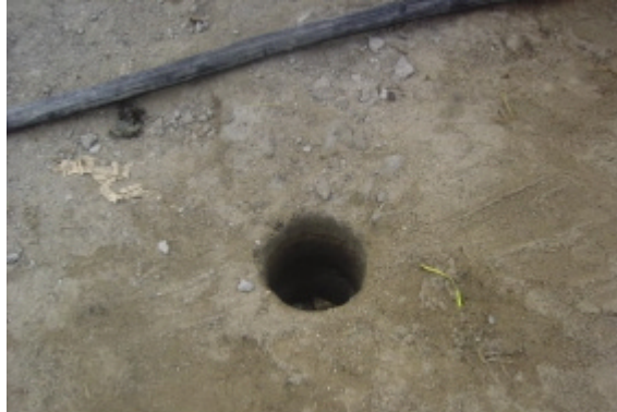
Photo 24. The execution of the holes for the anchor tie-rods
