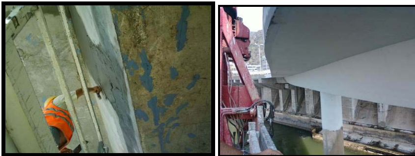
Fig. 13 – Repairation of the underside deck
