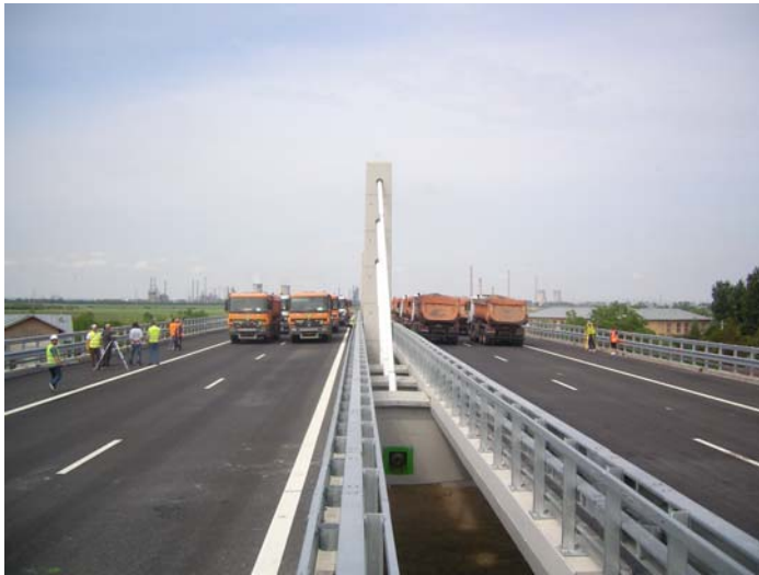
Figure 3. Anchorage of the harp in the RC transverse beams
