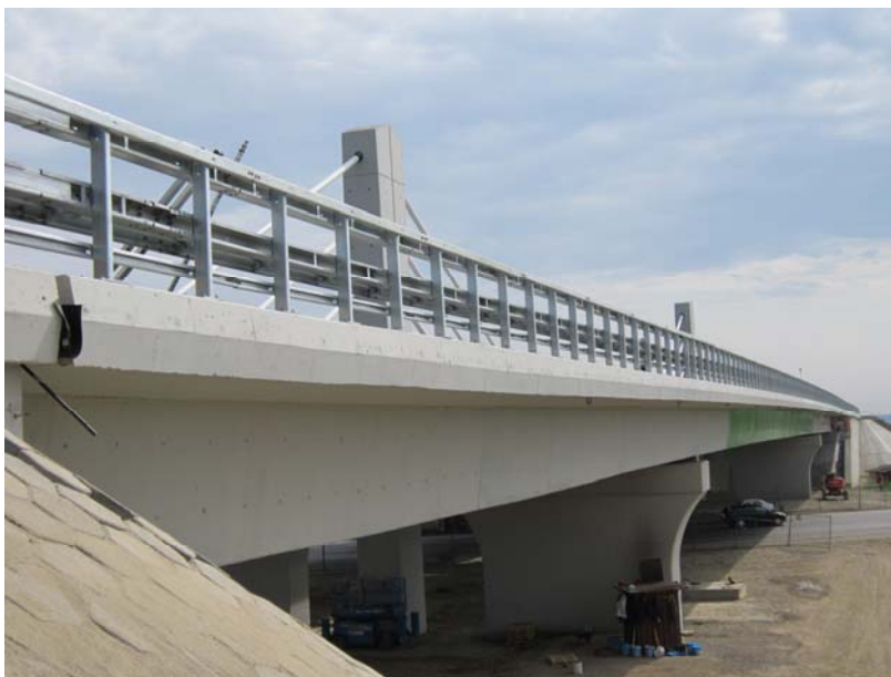
Figure 2. The 3 spans of 40,50m RC + 80,0m composite structure + 40,50 RC
