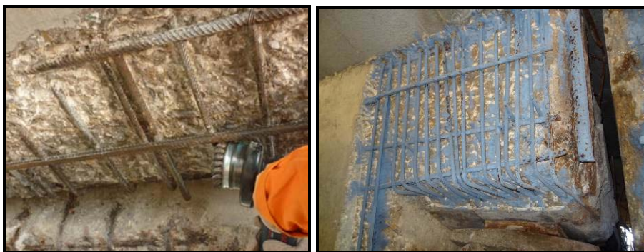
Fig. 6 – Reinforcement protection
