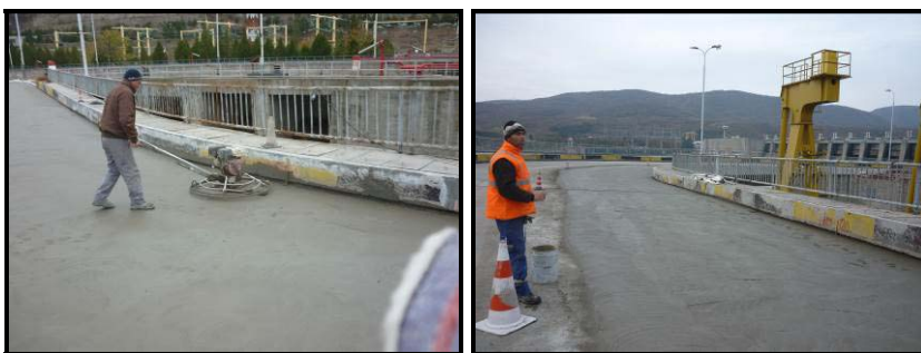
Fig. 13 – Execution of support concrete layer waterproof
