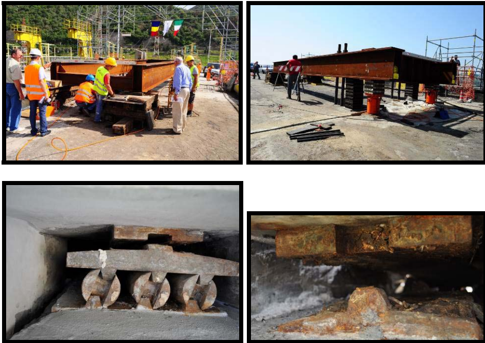
Fig. 11 – Lifting the independent deck
