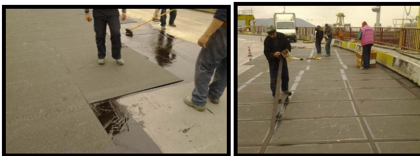
Fig. 14 – Waterproofing execution
