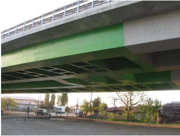
Figure 4. Anchorage of the harp in the steel transverse beams of the deck
