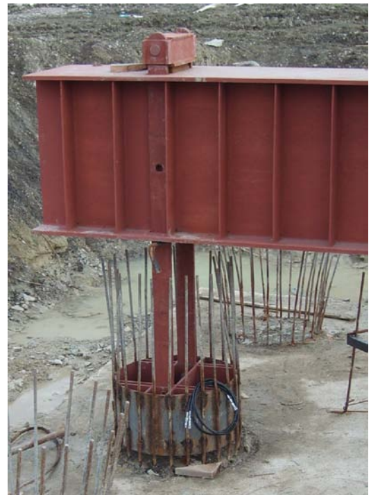
Fig. 2.3.2. Fitting the pile requested to pluck
